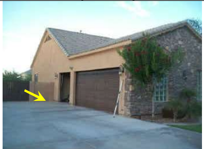
Photo 40: West driveway slopes to main home.
