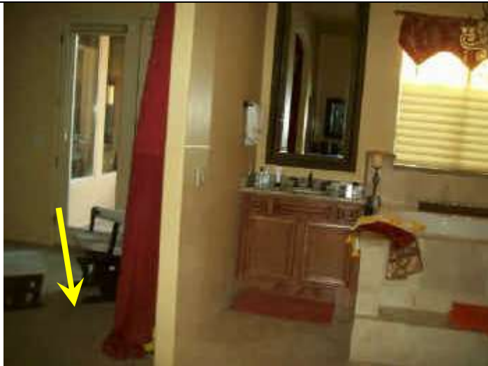
Photo 15: View looking west into master bedroom. Uneven flooring of carpet at entry to bathroom area.
