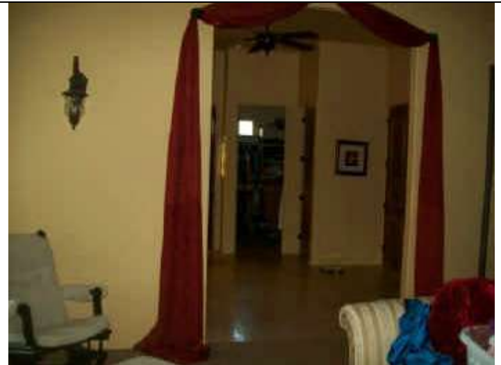
Photo 14: View looking north into master bedroom. Uneven flooring of carpet at entry to bathroom area.
