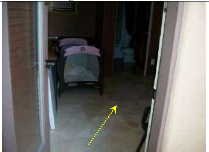
Photo 4: View looking west into guest room. Distress crack on floor tiles running diagonally through room.
