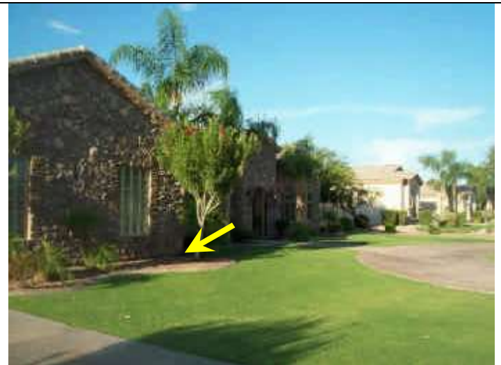
Photo 18: Front exterior view west end. Negative grade along stem wall.
