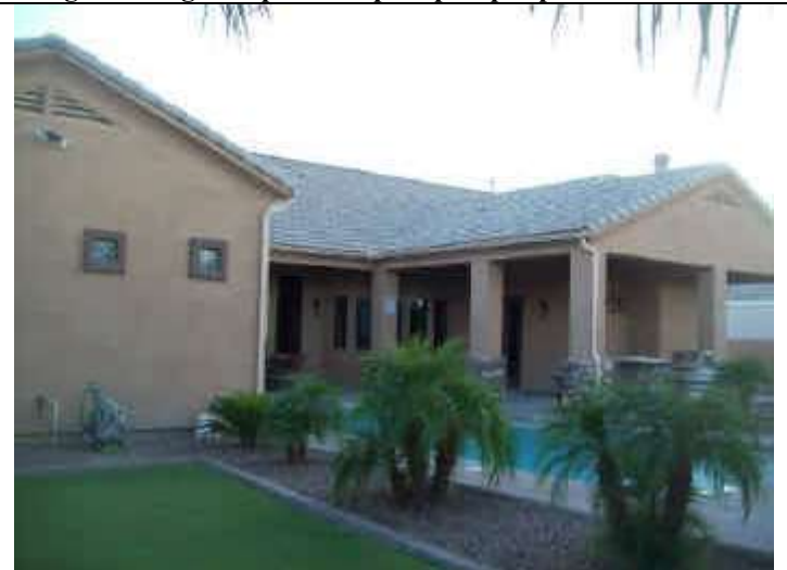
Photo 28: Rear exterior view.
